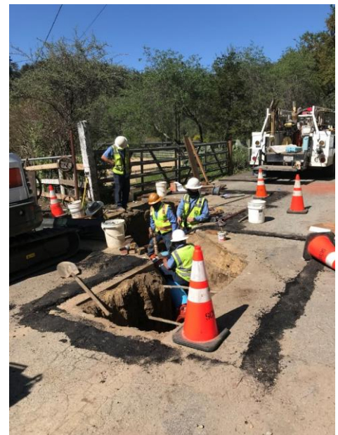
Water main replacement on OSE
