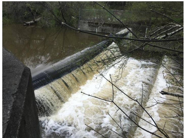
Felton Diversion Dam inflated and doing its job
