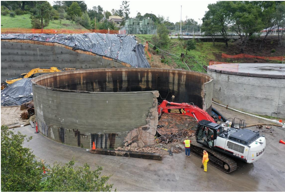
Concrete tanks demolition at the Graham Hill Water Treatment Plant, behind OSE
