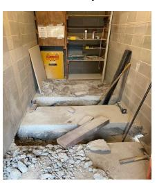
With CIP funds, Grant Park restrooms received a new sewer lateral and interior plumbing upgrade that has greatly improved the serviceability and function of the restroom facility. For years, staff had to close the restrooms periodically due to failed laterals and difficult maintenance requirements. Now the restrooms can remain open to park users and better serve the community.
