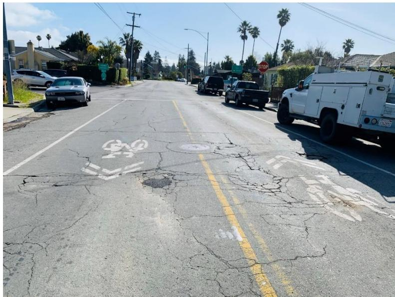
The 2021 Surface Seal Project is scheduled to start construction on May 24. The project, funded by Measure D and other funds, is rehabilitating several local streets with a single chip-seal and micro-surfacing.
