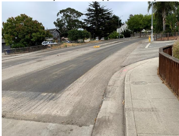
Overlay Project Cold In-Place Recycling at Delaware Avenue
