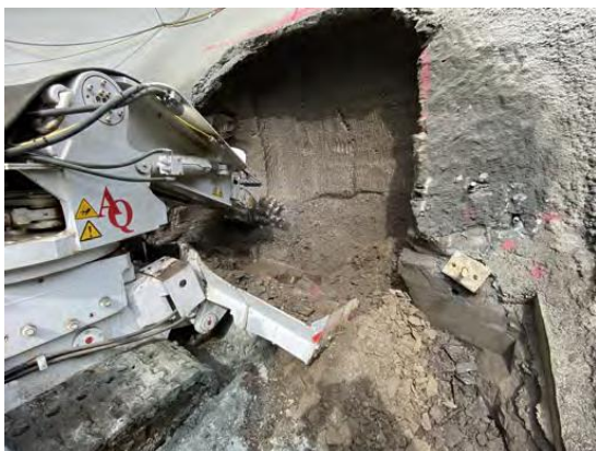
Photo of the tunnel excavation equipment
