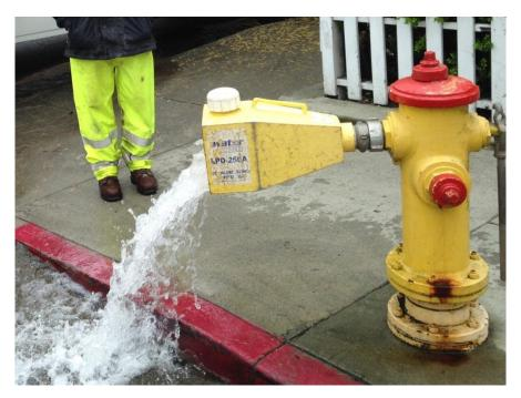
Flushing removes sediment in pipes and improves drinking water quality and lengthens the lifespan of the pipes. Flushing the entire system typically takes about 3-4 months. We'll only be flushing less than half of our system, so it won't take that long, but we'll be doing it sporadically so the public may see us
