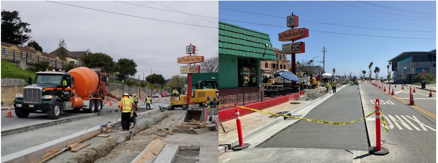
Pouring roadway PCC (cement concrete) Completed PCC, awaiting AC (asphalt concrete) top section
