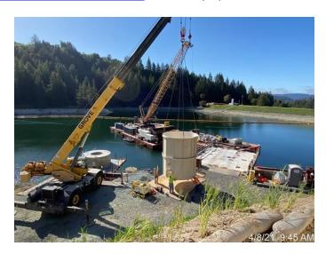
At the dam, tunneling progresses at ~10-12 feet/day. The in-reservoir work includes installing the foundations for the three, new, vertical, intakes. Each foundation consists of a concrete "donut" (see photo above) anchored into bedrock, and a steel debris wall that is bolted on top of the donut to protect
