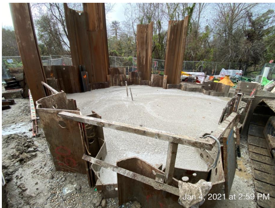
Receiving pit being backfilled to grade
