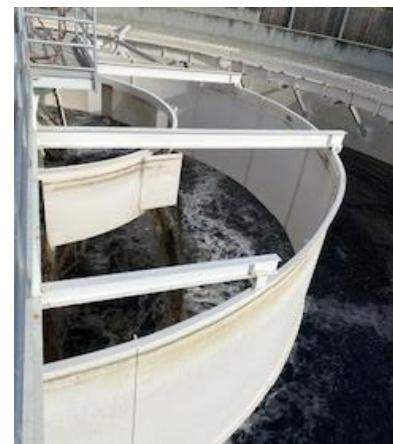
The “first flush” effect from this storm washed a large amount of heavy sediment out of the sewer collection system into the plant. One of the sludge thickeners was out of service for several hours at the end of the week due to heavy sand impeding the mechanical drive. By draining the thickener tank back to the headworks, operators brought the system back online as soon as possible and mitigated the negative impact all that sand would have on the anaerobic digesters.
