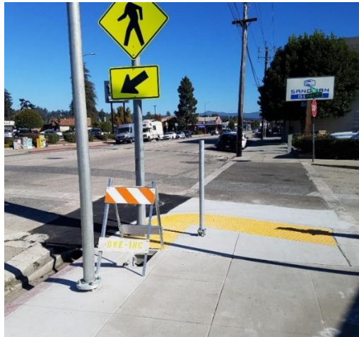
New curb ramp at the intersection of Soquel Avenue and Pine Street
