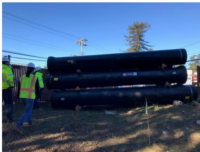
New 24" water main for the Coast Pump Station pipeline replacement project
