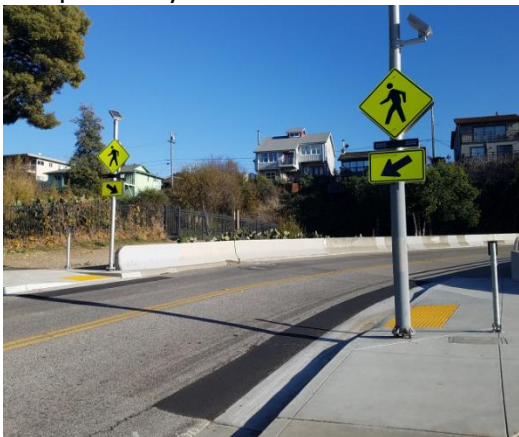
Lt: New rectangular rapid flashing beacon system at East Cliff Drive/San Lorenzo River Pathway (Lt) and Soquel and Mentel avenues (Rt.)
