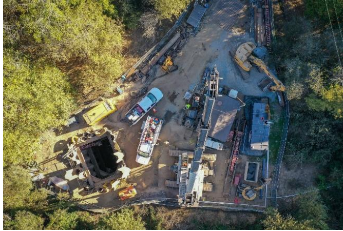
The receiving pit on Crossing Street, where the equipment will be demobilized.
