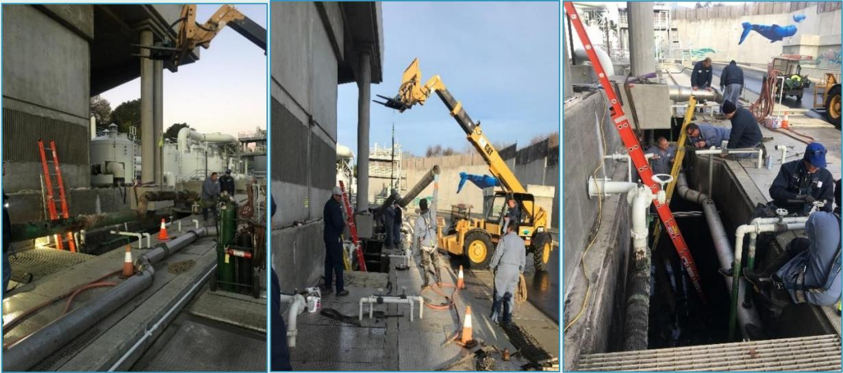
After the facility shutdown, we drained and cleaned the various flow 'temporary storage pockets' in the primary sedimentation basins.
