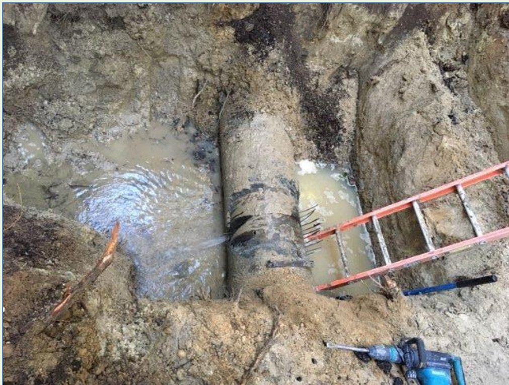
(Break on Newell Creek pipeline)
