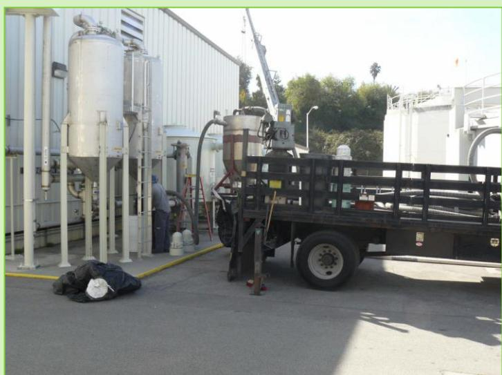
The carbon media was also replaced in two secondary foul odor carbon scrubbers. This activated carbon is generated from coconut husks. It removes sulfides and other foul air odors.
