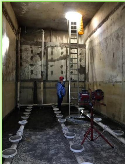
Operations drained and then entered the non-permitted confined space of Secondary Clarifier #2 to clean it in preparation for annual maintenance tasks.
