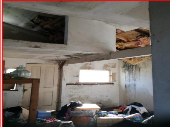
Unoccupied, unpermitted garage conversion with failing ceiling and visible mold
