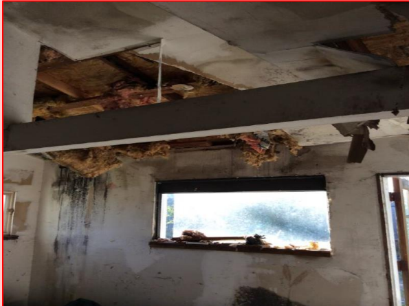
Unoccupied, unpermitted garage conversion with failing ceiling and visible mold
