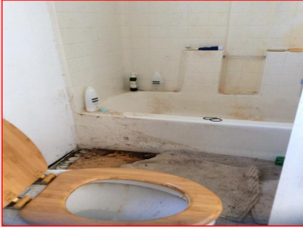
Failing subflooring in the bathroom
