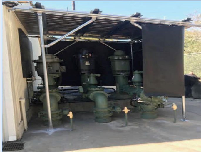
(Pumps with new noise canopy installed)
