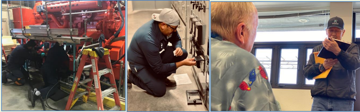
Mechanics and contractors rebuilding Cogeneration Engine #2. Operator removing paddles from Cogeneration Engine #1 control panel, part of the Stand-Alone Test. A recently retired operator received a recognition of service plaque.
