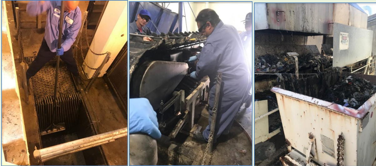
Operator raking an influent channel. Mechanics replacing barscreen conveyor bearings. 'Hopper' used to collect rags removed by the barscreen while conveyor was being repaired.
