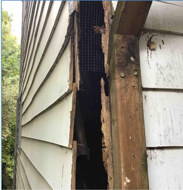
Corner of house framing as seen from the outside has completely deteriorated. See next picture from inside.
