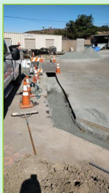
Electrical Feed Installation
