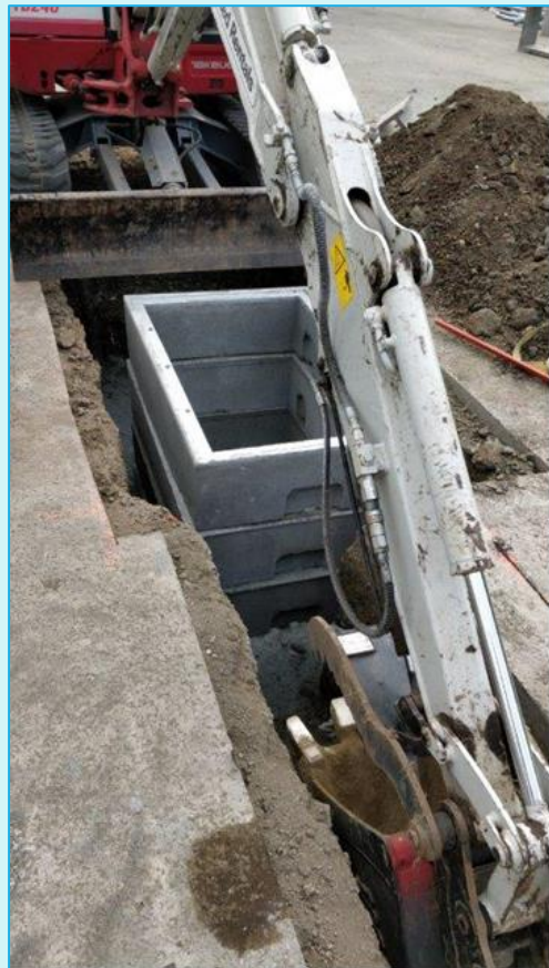
Electrical Feed Installation
