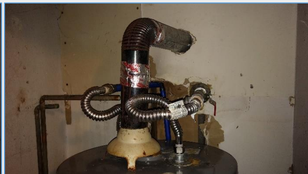
Improper venting and strapping
