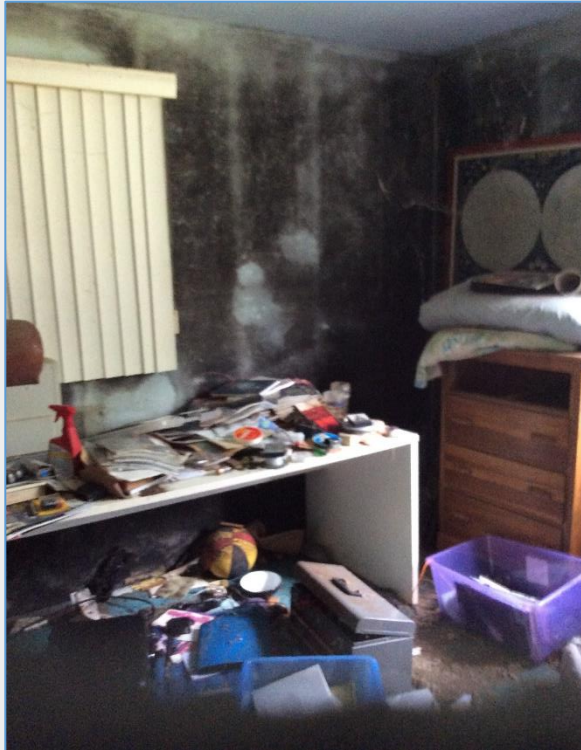
Bedroom has mold going up to the ceiling that should have been blue paint
