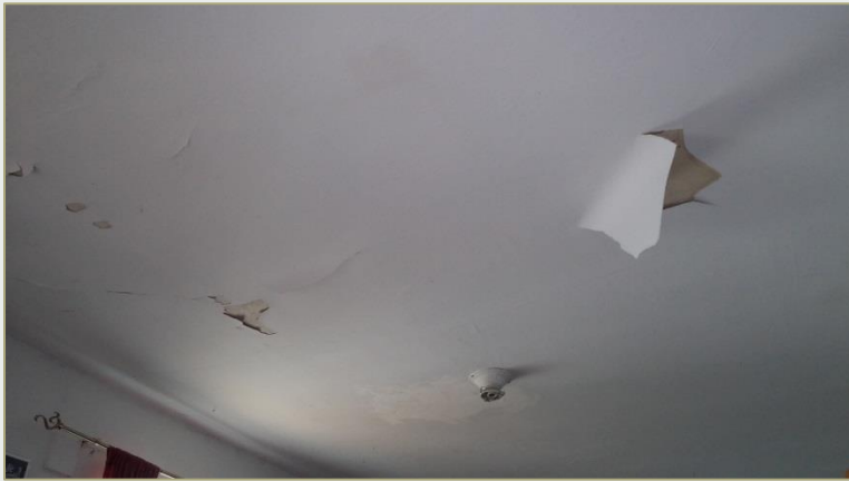
Water intrusion in this bedroom area has caused drywall in the ceiling to sag and peel
