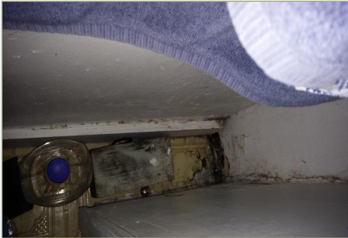
Dilapidated flooring due to leaky fixtures and pipes, can cause mold and deterioration of the subflooring
