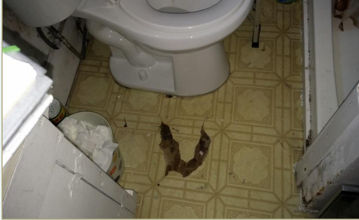
Dilapidated bathroom flooring due to moisture
