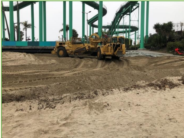
Building berm to prevent river from taking over Main Beach
