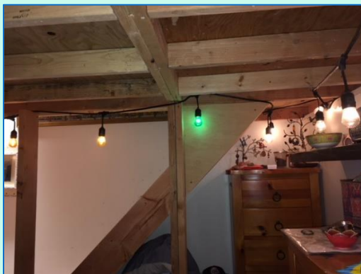
Substandard stairs and loft area without permits
