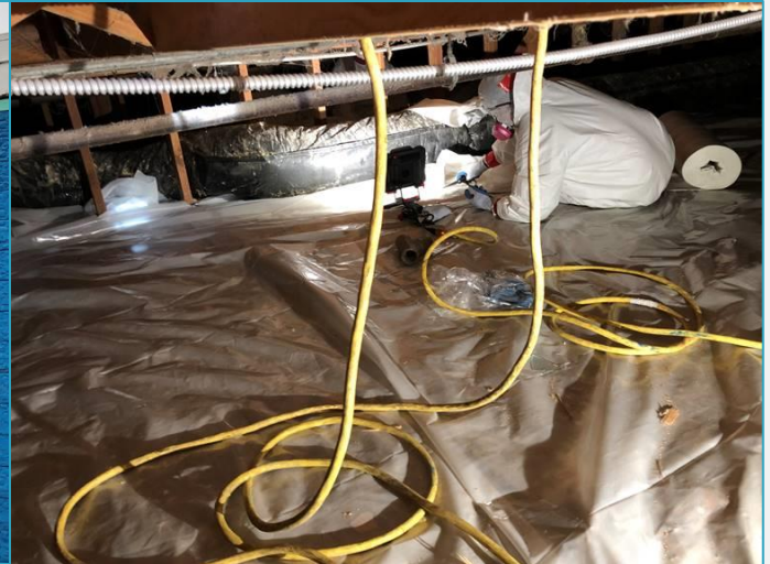
Installation of protective sheeting under the building to capture runoff and debris.
