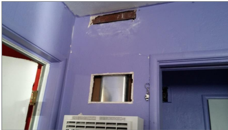
New gas wall heater installed without permits and in an unprofessional manner creates a possible fire hazard.
