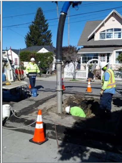
Leak repair on Washburn
