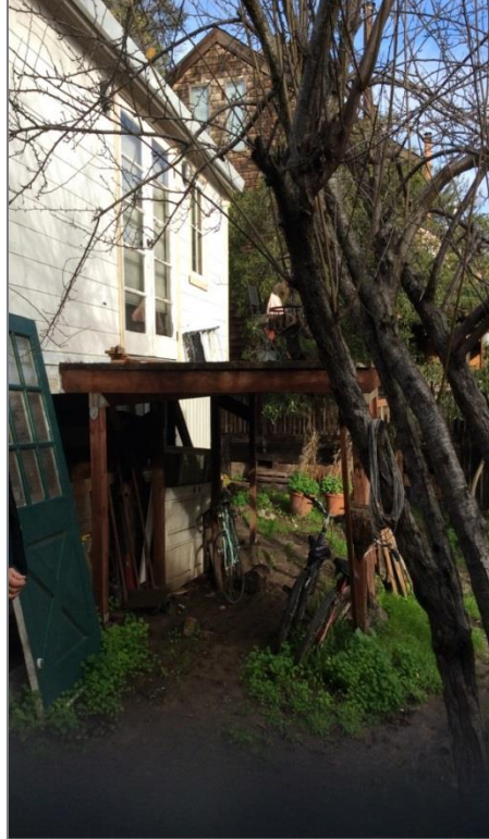
Unsafe, illegal construction of an elevated deck with no safety railings.
