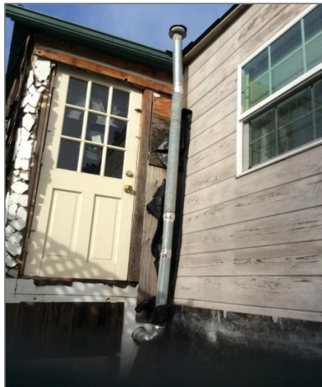
Unpermitted addition – door leading to fall hazard since no exterior stairs are present and unsafe venting with possible fire hazard.
