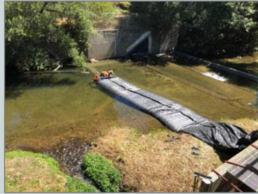
Laying out the new AquaDam
