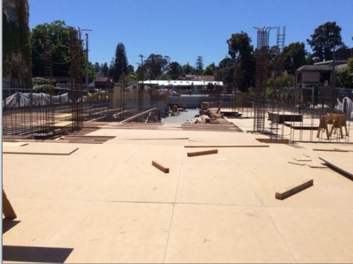
Photo 3: Plywood support and framing for street level.
