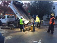
Tuesday afternoon a contractor boring on Center Street hit a hydrant lateral pipe causing quite a mess. (Fortunately it was a 6" pipe so the water loss wasn't significant.) The valve that controlled flow to the hydrant was in poor condition, forcing us to do a repair that night. After repairing about 4 feet of pipe and returning the main to service, another leak presented itself on the valve for the hydrant. Repairs and cleanup continued through the night.
