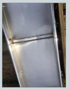
The metal slide at Ocean View Park has reopened. It was temporarily closed for repair due to safety concerns. Extended use of the slide had worn the metal thin. Metal patches were welded to the slide in order to strengthen and pro-long its lifetime.
