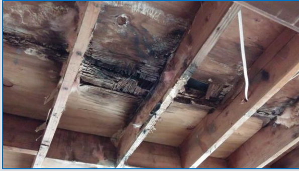
Inside house - Leaking roof destroyed ceiling
