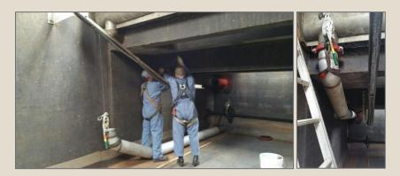
Maintenance has been tackling Clarifier 2 annual inspection and repairs which includes replacing the old corroded sluice drain gate with a stainless steel one. The original cast iron gate (photo below on the Left) was in use for 20 years, we can see the corrosion rate is pretty high. The new stainless steel gate (center photo) has a life expectancy of 100+ years and has
