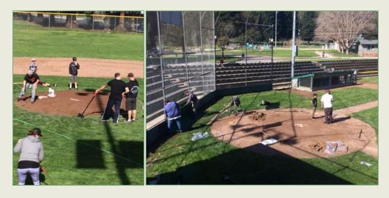
De Laveaga Park batter boxes received an overhaul with the installation of clay bricks that will stop players from digging deep holes into the ground. This was identified as a safety issue while softball players were running home. The repairs were completed in time for the kickoff of the adult sports programs.
