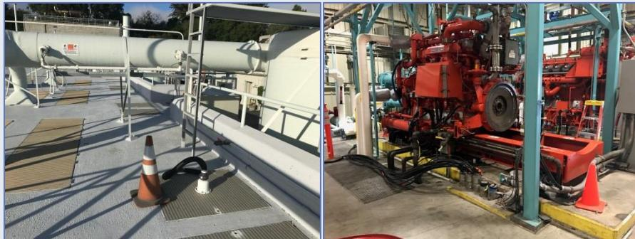
Work by operations, maintenance and electrical staff has begun on upgrading the Tunnel Portal Box (TPB) to accommodate bioassay equipment. The first photo below shows the temporary installation of an alternative pH and chlorine residual stilling well, to ensure we still meet permit requirements while the permanent TPB is upgraded.
