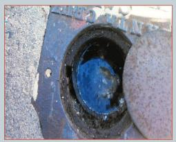
Sheen visible in sewer clean out after spill
