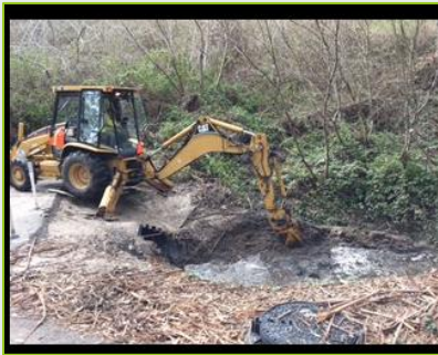
The wastewater mains crew cleaned the Lombardi Creek storm drain outlet structure.
