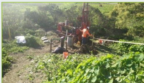
Completed replacement well (medium and shallow probes inside) and drill rig.
