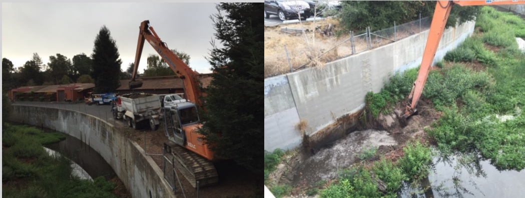
October 22, 2015: Sediment removal from Branciforte Creek Channel.
