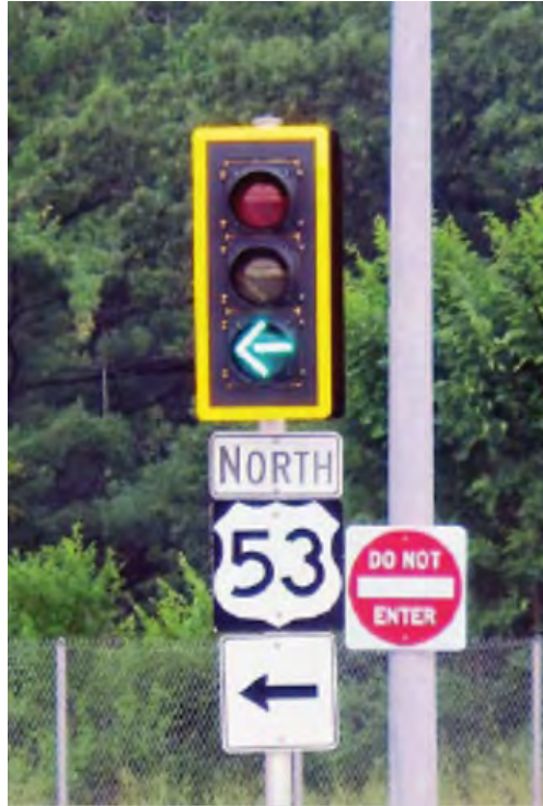
Figure 21. Example of Signal Head with Retroreflective Borders along Backplate
