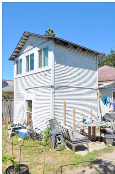
Figures 3 and 4. Left image details the rear elevation's shed, which has been converted to living space. The original cottage was attached to a rear outbuilding before 1950 and the second story added. Right image details the rear elevation.
