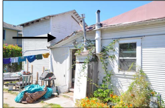
Figures 1 and 2. Left image shows the front (north) and right side (east) elevations. Windows, doors and roofing material have been replaced. Right image details the east elevation where the rear outbuilding is connected to the house with a poorly constructed shed roof (arrow).
