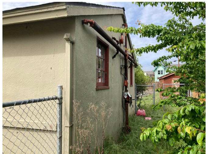
Figure 4: Figure 5: North façade, looking west.
