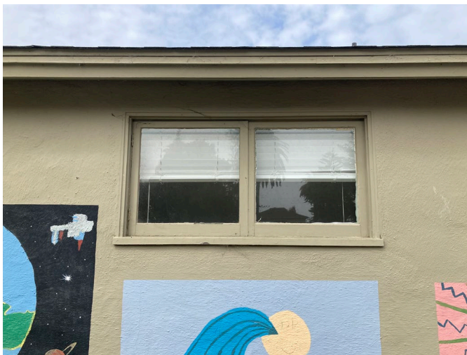
Figure 3: Typical wood casement window at the east façade, looking west.
