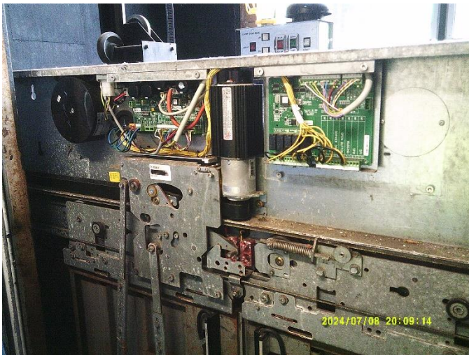
19. Linear door operator with control circuit boards exposed.
