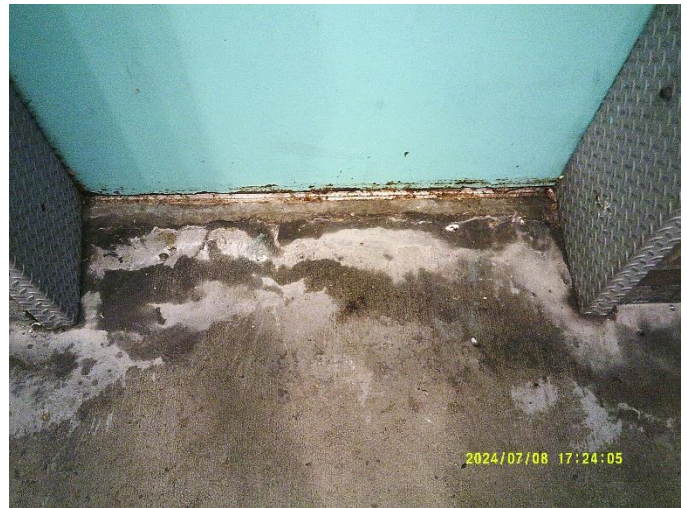
2. Evidence of water pooling at the opening
