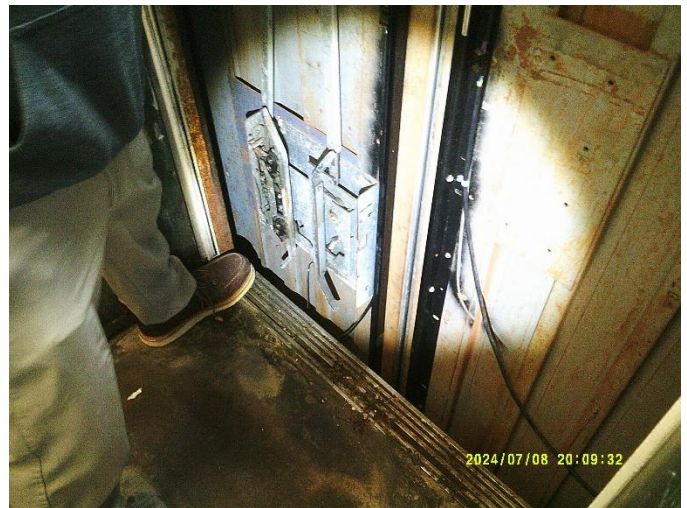
20. Car doors, detector strips and door clutch as seen from landing with car slightly below level.
