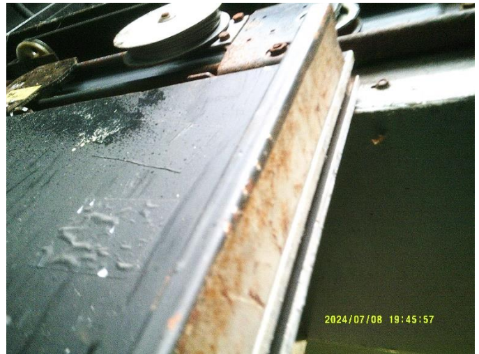
18. Entrance/landing elevator door panel rusted.
