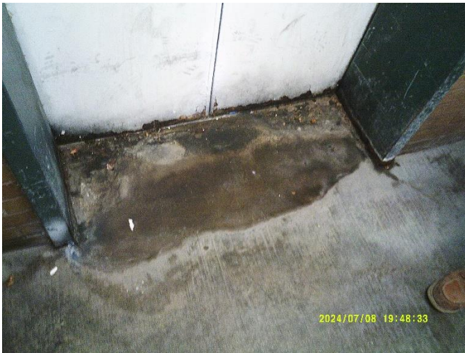
13. Street/Ground level entrance with evidence of pooled water.
