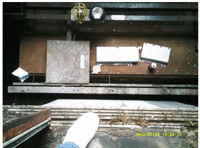
16. Car canopy rusted, as seen from upper landing.
