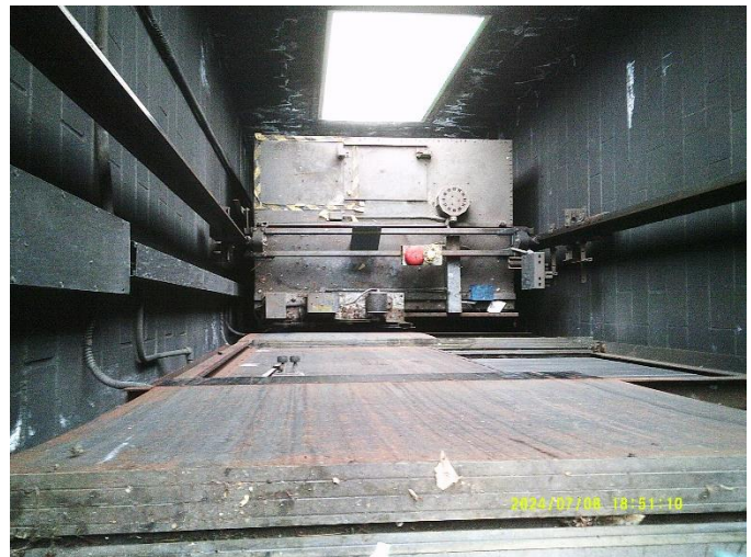
12. Top of car seen from opening at upper level.
