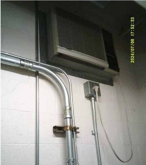
5. AC unit mounted directly above mainline power.
